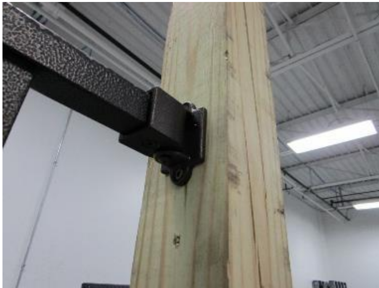
Photo No. 9 Top Rail Bracket Installed In-line
